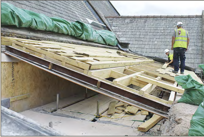
Building the replacement wooden framework in progress.
