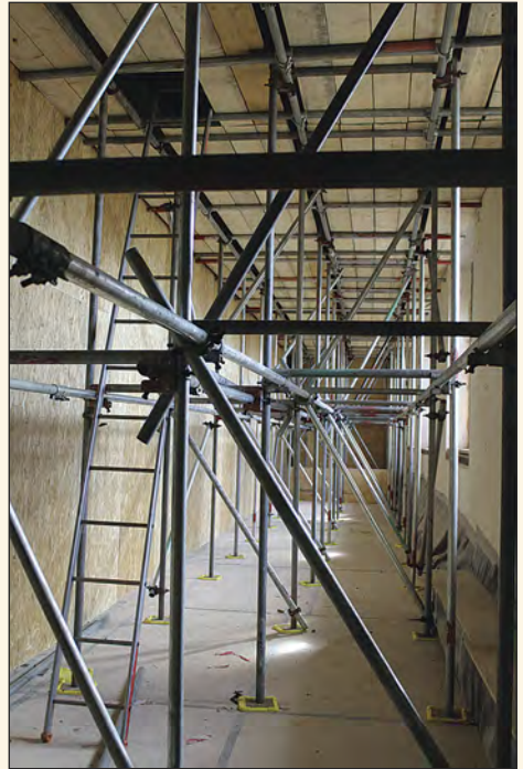
Internal high level platform to catch the concrete rubble.
