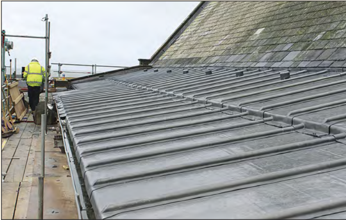
Re-clad roof. Leadwork nearly completed.
