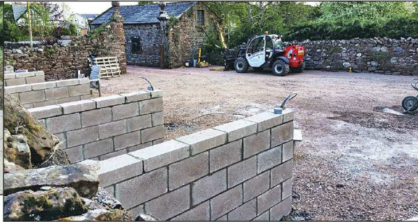
Alcoves under construction.
