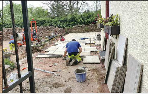
...and patio being paved.
