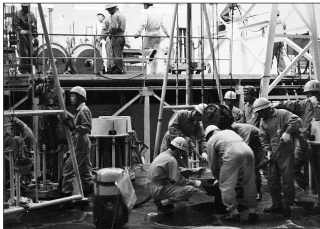
Reactor during fuel loading.
