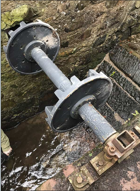
Shaft resited by R J Slater ready for timbers.
