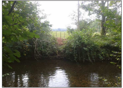
The hole where the bridge used to be. Carolyn Sayers
