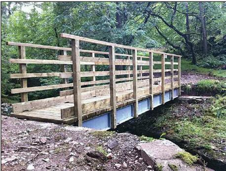
The second is a new bridge across Scalderscew Beck which provides convenient access to the other side of the forest. The bridges are installed along the route of the old forest road, allowing re-use of existing abutments. This meant that construction was relatively quick, despite the heavy rain during the construction period. These photos, taken by Trevor Brown, show the bridges during their construction.
