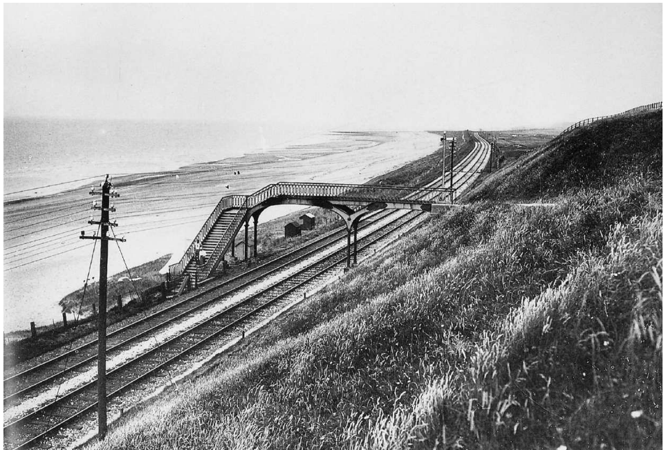
From a camera position north of Seascale station the main line is seen following the coast, in a northerly direction, towards Sellafield. On its way it passes beneath an attractive cast iron accommodation bridge carrying a footpath over the railway from the village to the sea-shore. As with the bridge at Ravenglass station the Seascale footbridge has no railway connection, but in common with all bridges that cross the railway it is allocated a bridge number, in this instance 161. The crossing still exists, but the illustrated bridge has been replaced by a different structure.
