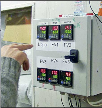
Mark explains the processes and components involved in fermentation, including the critical temperature control at every stage.
