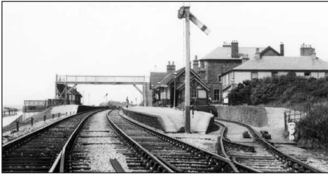
The Seascale signalbox and cross-over track that gave access to the goods yard on the east side of the main line. The suspended curved bracket on the right was to ensure that wagons leaving the goods yard were within the permitted loading gauge. ▼
