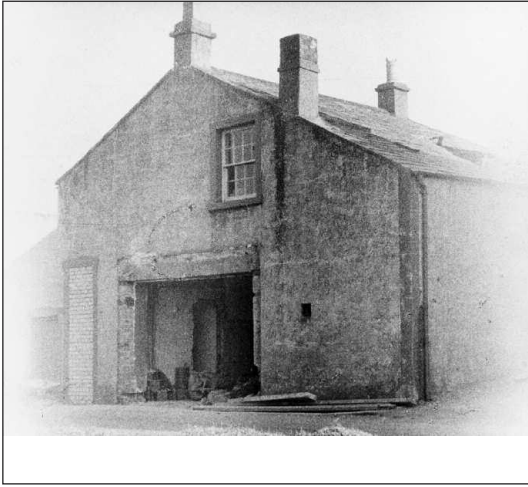
1958: Top Shop during conversion.
